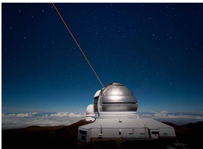
Nighttime image of the Gemini North Observatory. The laser beam produces an artificial star in the atmosphere of the Earth which is used as a reference star for the adaptive optics systems.
